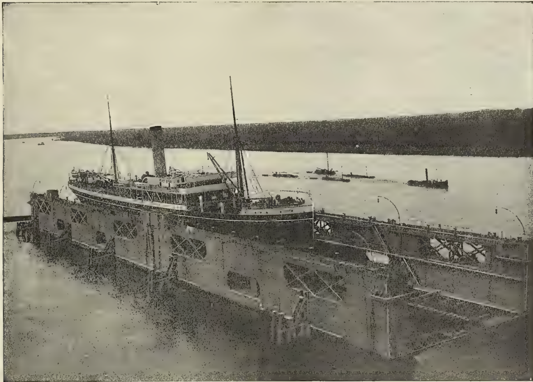
THE FLOATING DOCK IN THE OUTER HARBOR AT COPENHAGEN.
